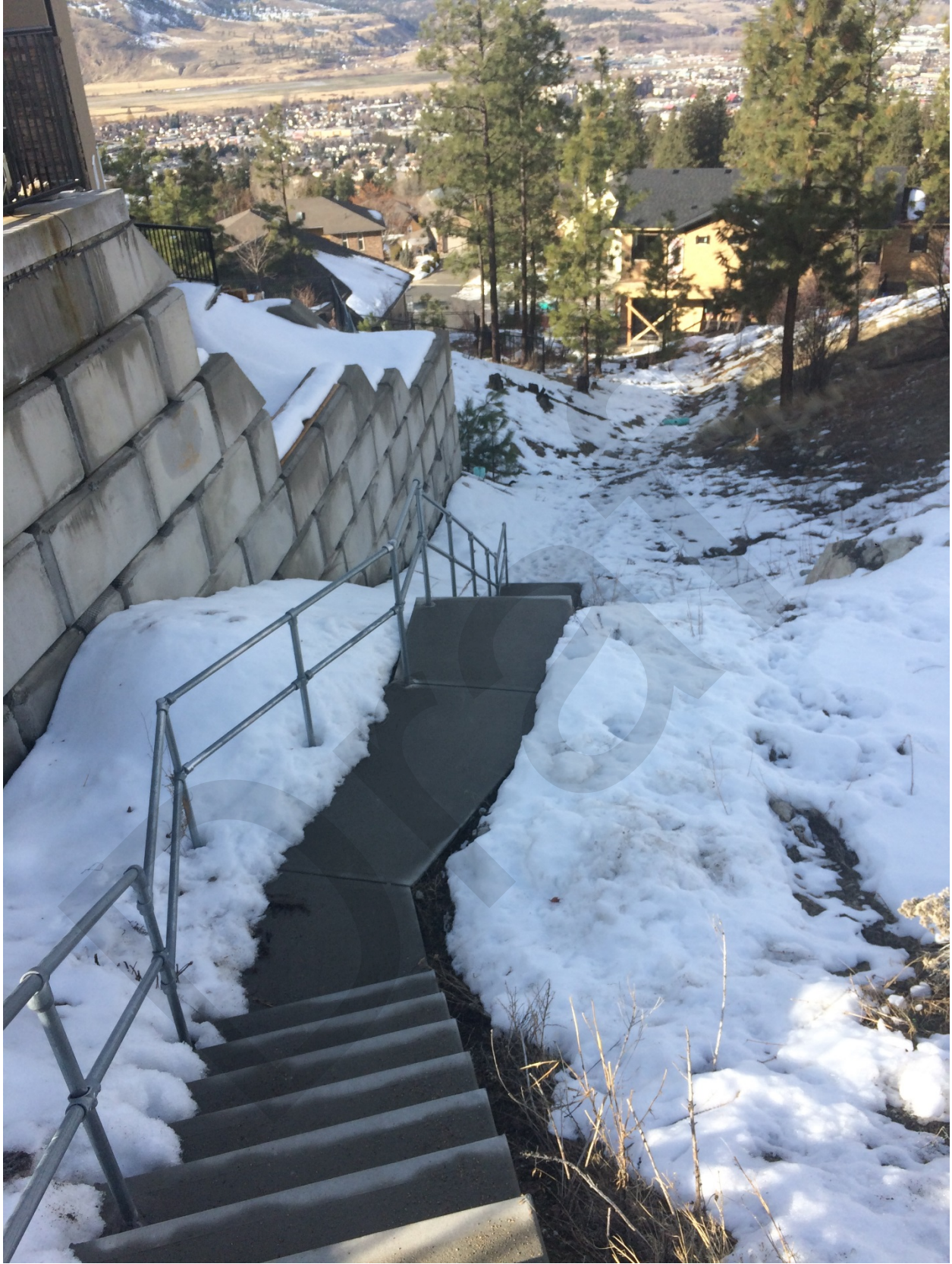
Figure 1: Image of public walkway looking west with existing over-height retaining wall on left. Similar wall is proposed on right.
